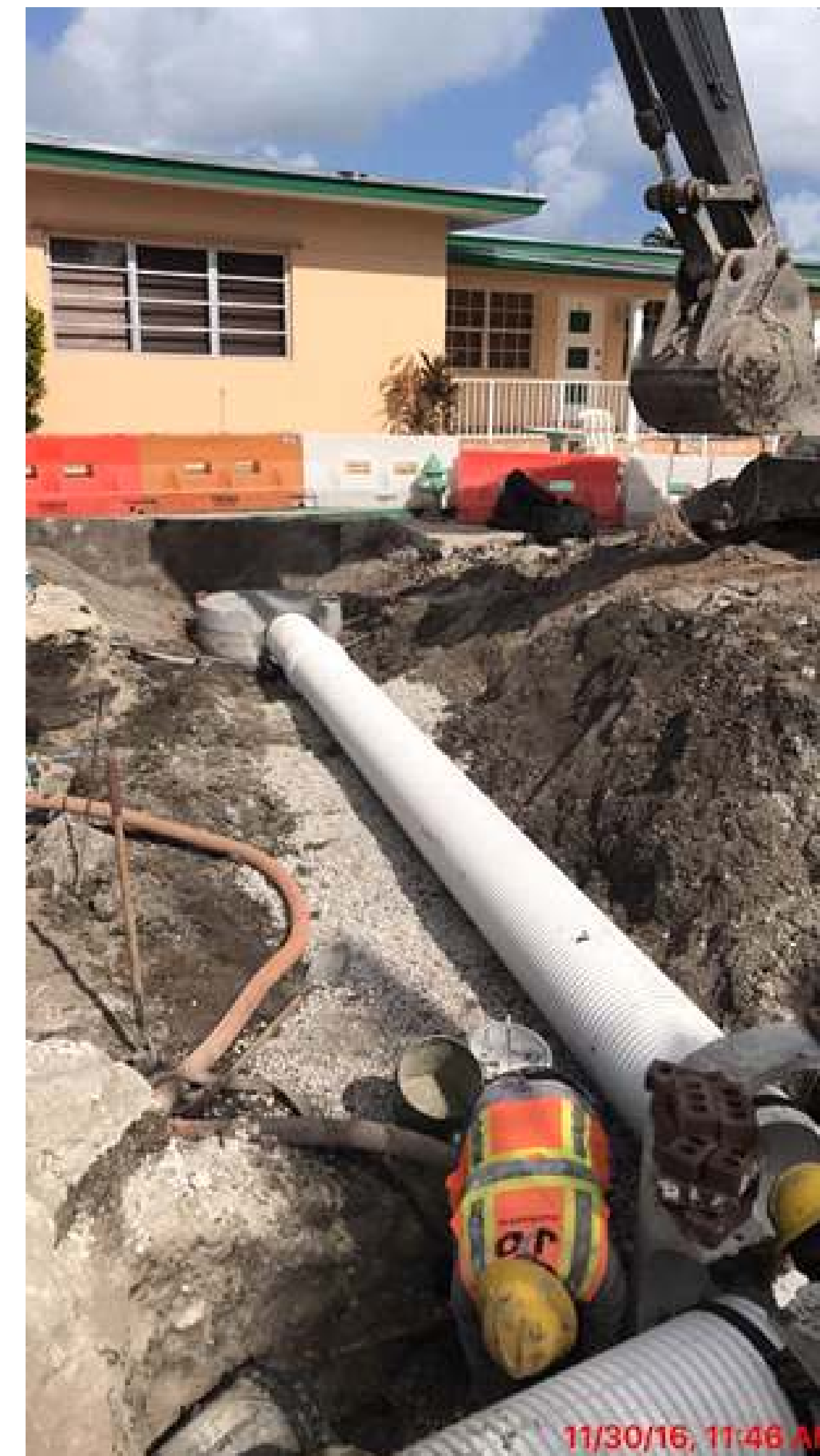
Typical Storm Drainage Installation
