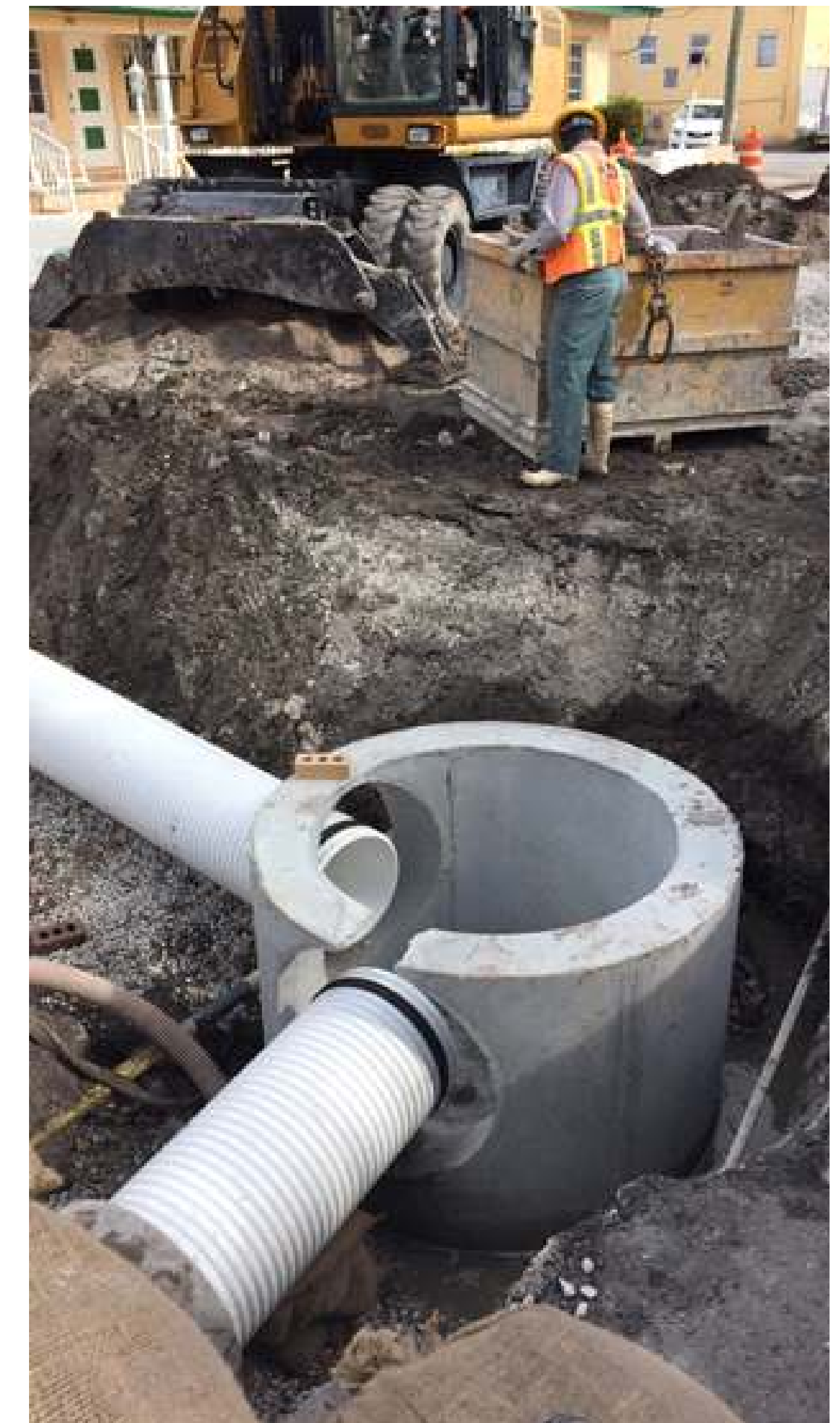
Typical Storm Drainage Installation
