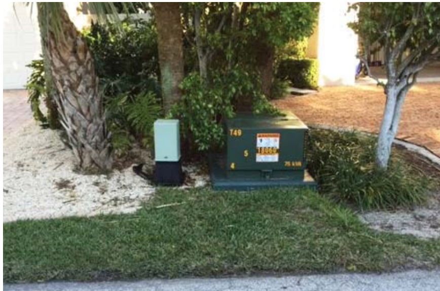
Figure 2: Example Easement on Private Property (before landscaping)
